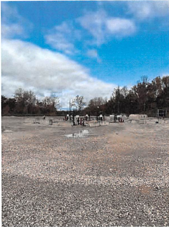
Erlewine Well Pad Site
