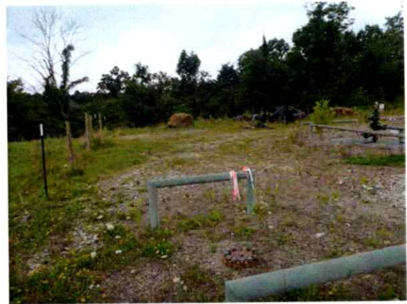
Well Pad Site (West)
