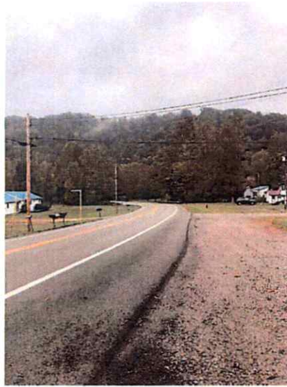
Willey #1 Access Road Approach
