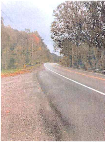
Willey #1 Access Road Approach
