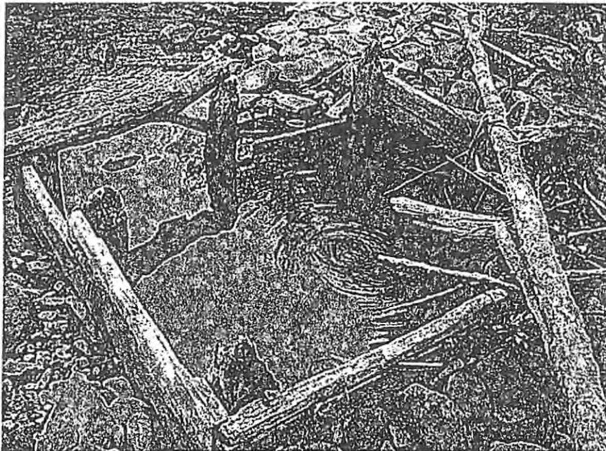
Randolph 106/BW-1 well bore in Glady Fork on July 7, 2005. Well bore has a gas discharge, also small amounts of oil produce sheen on the water inside and outside the wooden cellar.
