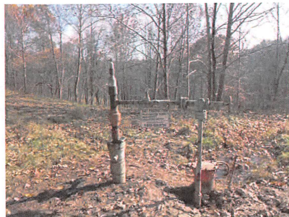
WV 460671 Well Pad Site (Looking East)
