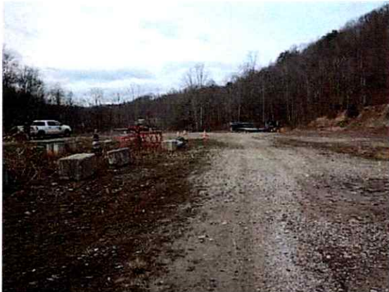
Jones Pad Entrance
