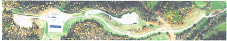
Site is fully stabilized.
