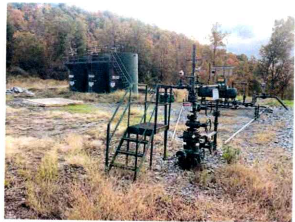
L-005686 Well Pad Site
