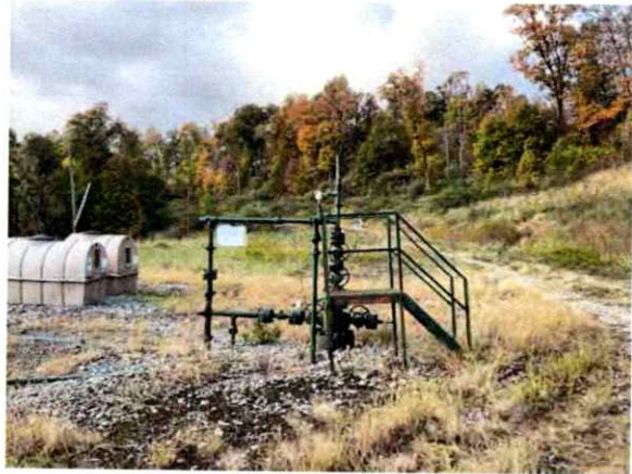
L-005686 Well Pad Site
