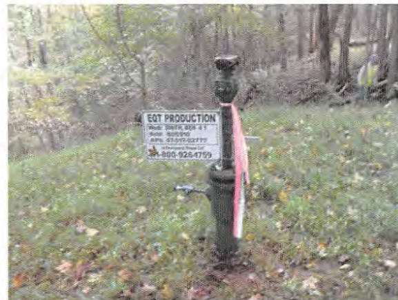
WV 605510 Well Pad Site
